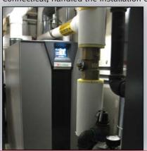
the new system. Due to the small size of the mechanical room, removing and replacing the boilers within the tight space posed a slight challenge. The existing boilers occupied a small footprint and were PVC direct vented, which SYNC was able to align with seamlessly to simplify the installation. "It was a really tight fit in the mechanical room, but SYNC's compact size and direct vent design was the perfect match for this replacement," said Montas.
